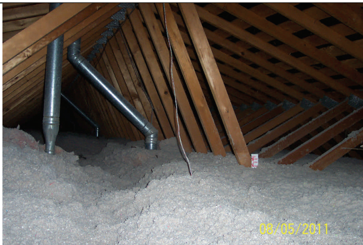
The attics are now insulated with approximately 13" of R-50 cellulose loose-fill insulation
